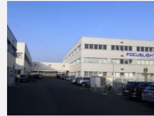
Dortmund, Germany Operation Center
