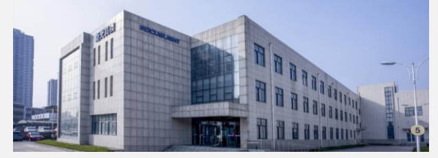
Xi'an, China Focuslight HQ, Operation Center
