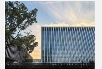
Haining, China Hefei, China Operation Center (being constructed)
