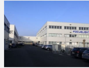
Dortmund, Germany Operation Center
