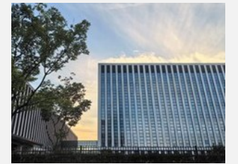
Haining, China Hefei, China Operation Center (being constructed)
