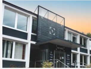
Neuchâtel, Switzerland Operation Center
